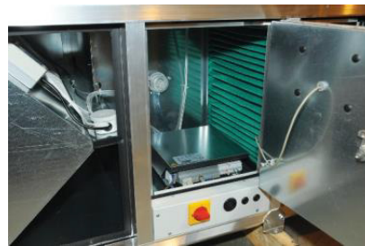
Interior view of technical compartment "EASY" controller
